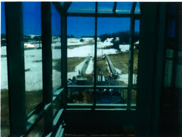
Figure 7: Existing glazing to be upgraded
