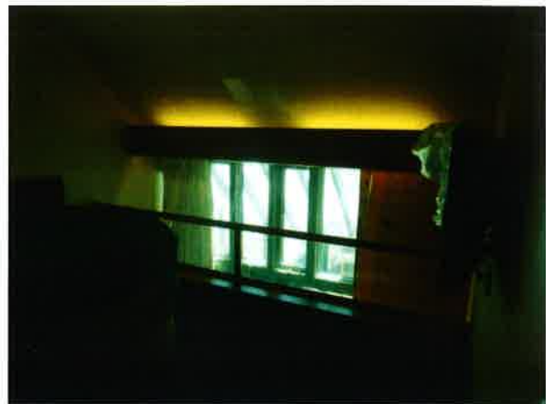
Figure 8: Curved ceiling to be removed and replaced with new raking ceiling + master bedroom extended into the void
