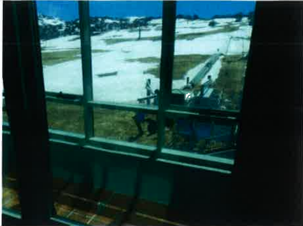
Figure 5: Existing balcony to be converted into a kitchenette
