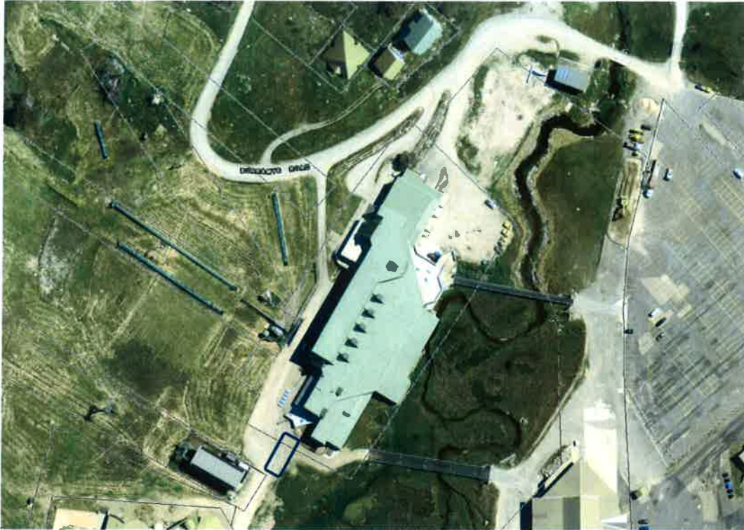
Figure 3: Suitable Material Storage Area
