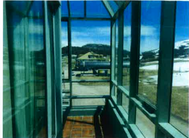
Figure 6: Existing balcony to be converted into a kitchenette
